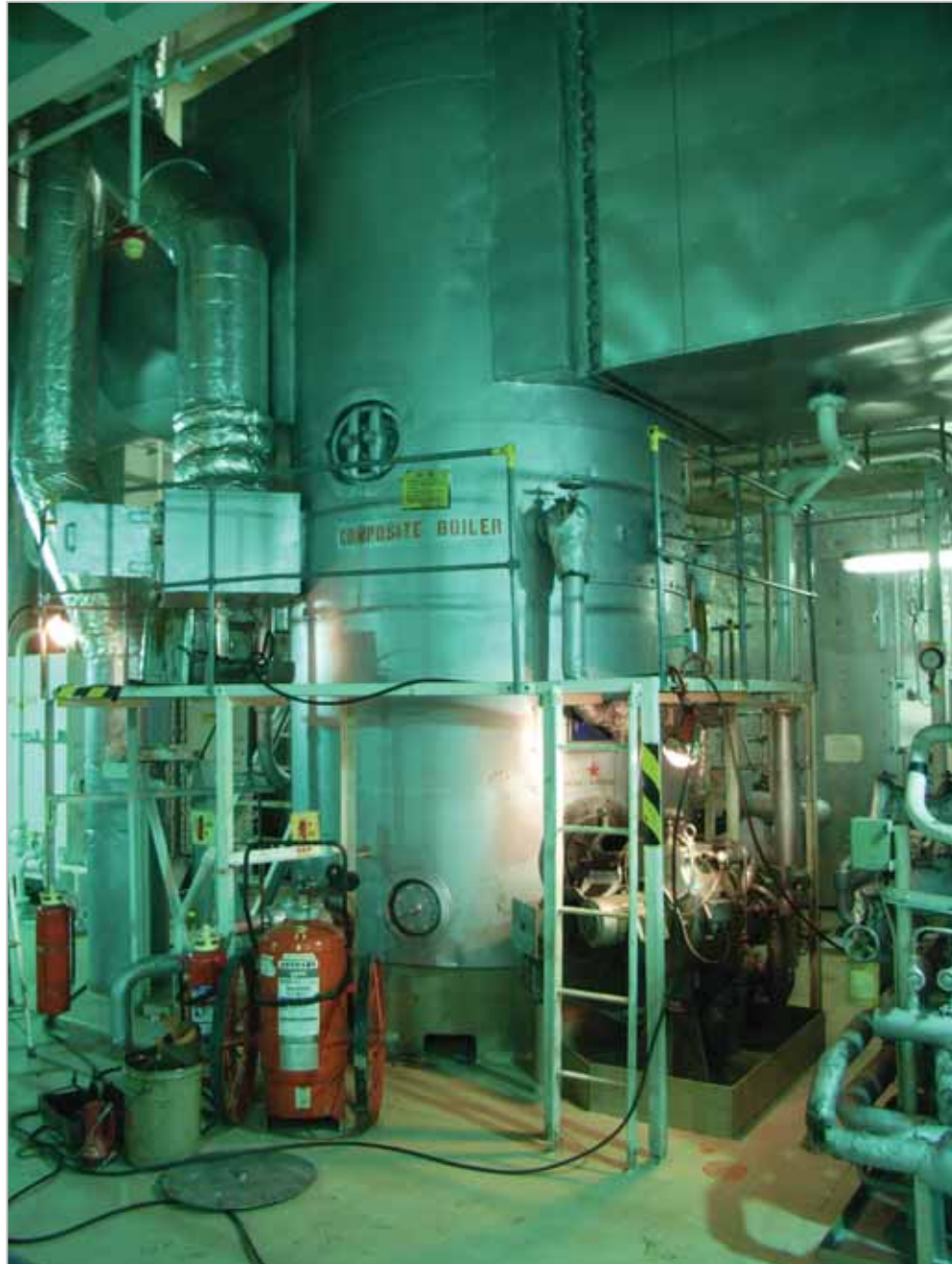
Figure 2: Shirane's composite boiler
